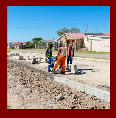
The workers have begun installing kerbs on the section between Extension 4 and Joza, however, the recent heavy rains have delayed the project.
